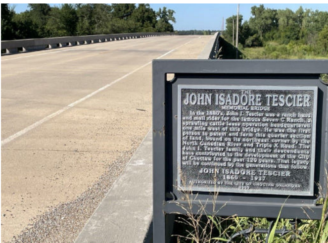
The John Isadore Tescier Memorial Bridge
