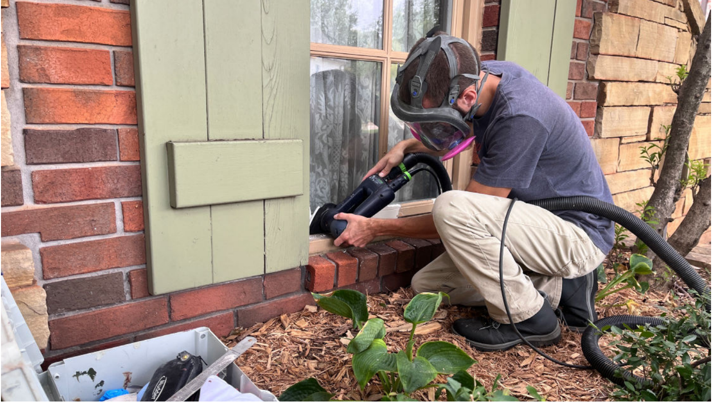
Blake Elwell repairs a window frame using Preservan technology.
