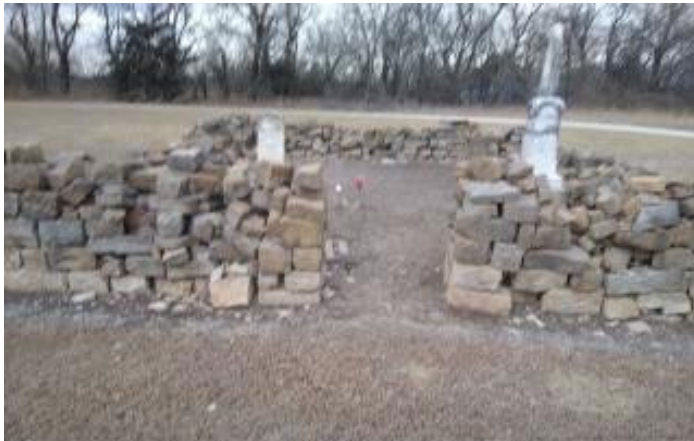
East Wall Before
